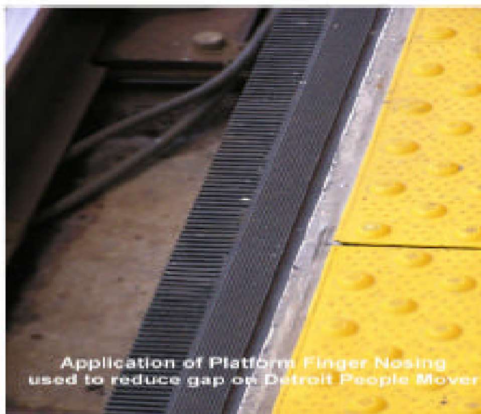
Figure 5. Extended rubber fingers on platform edge gap filler.
